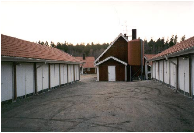
Fig. 32 - Garages off commonhouse
