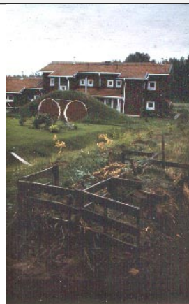
Fig. 6 - Small windows on North side [Bokalders 1995]
