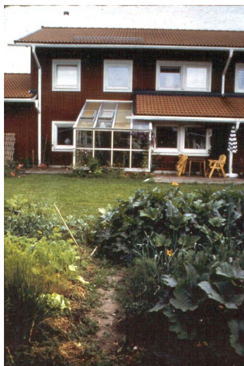
Fig. 4 - South Facade & Garden [Bokalders1995]
